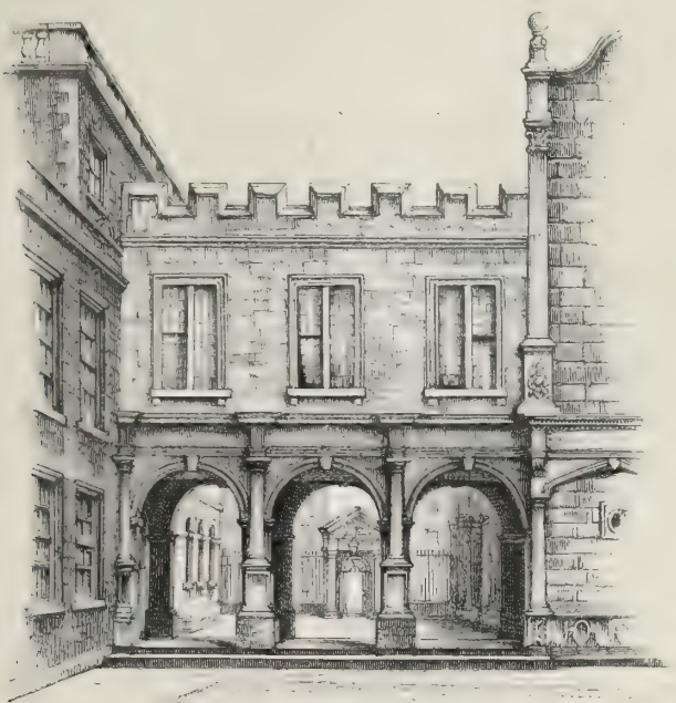
Fig. 15. North Cloister, as rebuilt in 1709.
